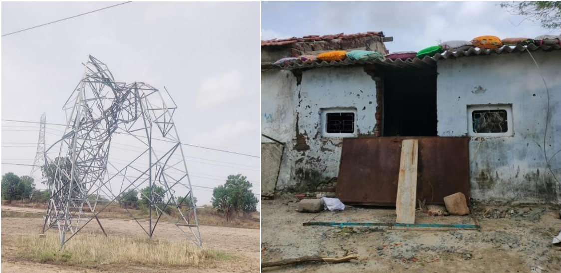
Pic 2 and 3: Damage to electric pole in Jangi (left), Damage to door in Surajbari (Right)
